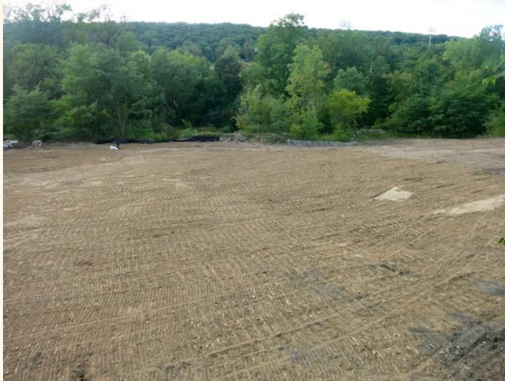
Cleared Site (Fall 2016)
